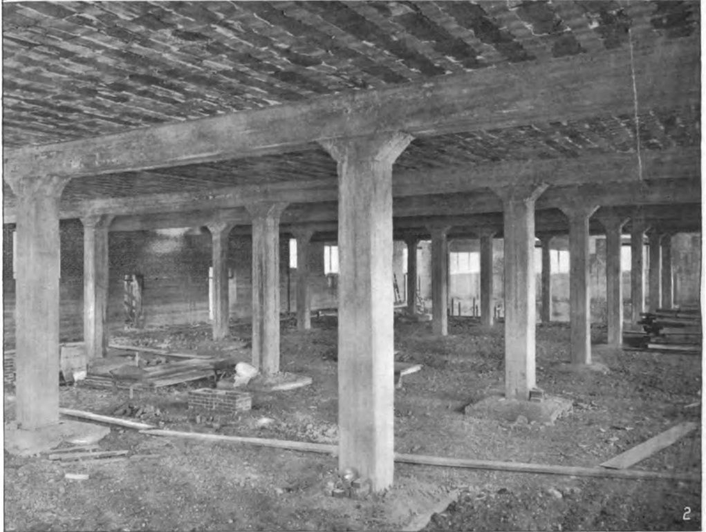
2 Reinforced Concrete Hollow Tile Rib Floor Construction
