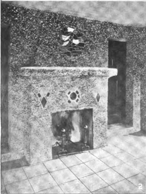
1 Glens Falls Bridge, Arch of Concrete, with Spiral Stairway 2 Fireplace of Concrete with Selected Aggregate and Inlaid Tiles
